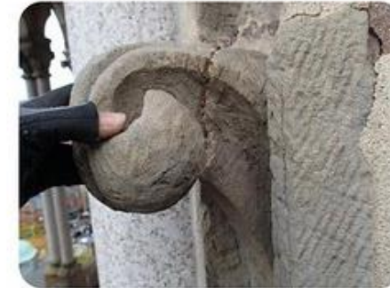
☞ Repair Cracked Ornamental Stone (Crocket)
