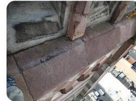
☞ Repair Joints between Stones
