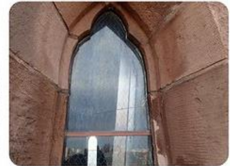
☞ Replace Cracked Glass
