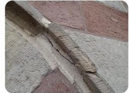
☞ Repair Sandstone Spall
